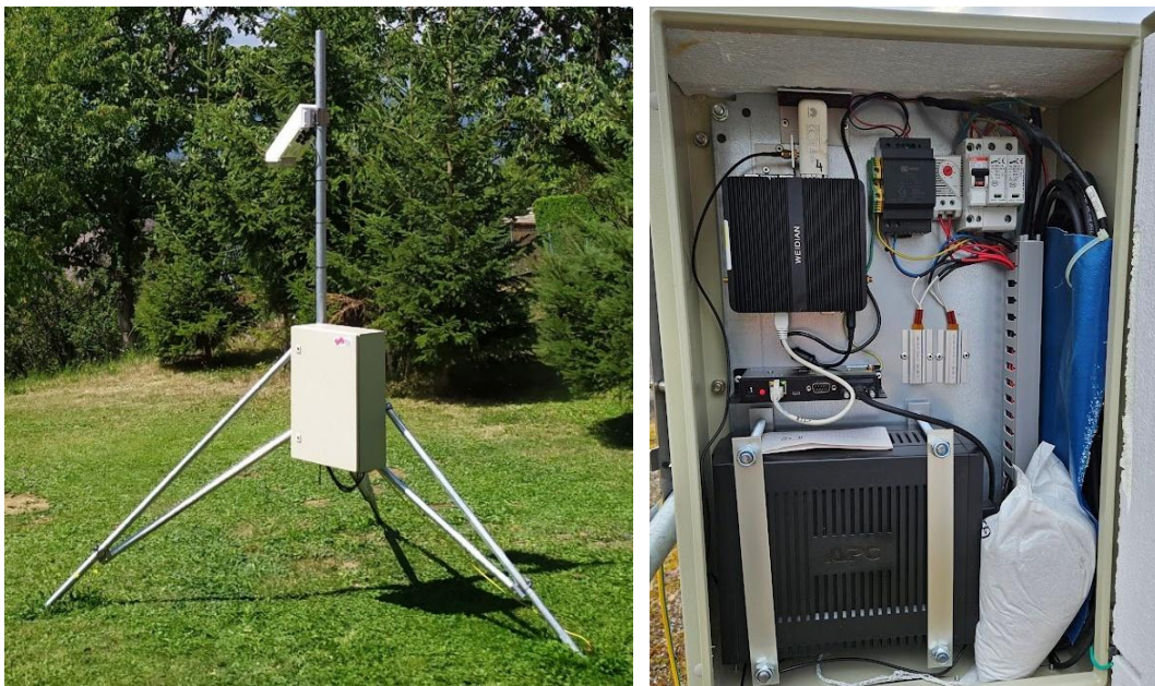
Figure 12: Tripod with mounted FM-sensor and control box (left), equipped control box with peripheral devices (right).
