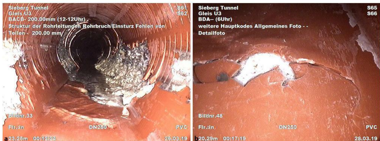
Figure 2: Camera inspection after intensive cleaning processes in the Sieberg tunnel - complete destruction of the pipe wall (a), or local destruction of the drainage layer after intensive mechanical cleaning (b).
