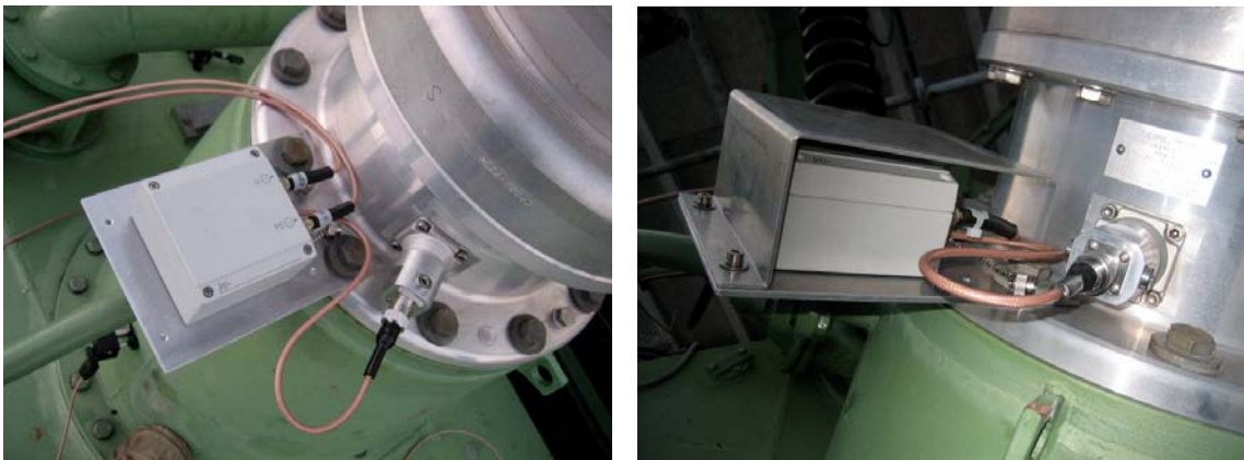
Fig. 7.41 Bushing tap adapter BA and bushing coupler unit BCU on a Micafil® bushing
