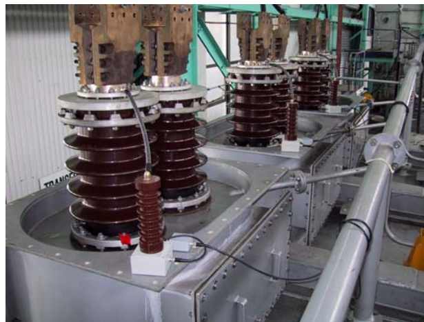
Fig. 6.17 Coupling capacitors with RF CT used on LV bushings of a GSU transformer.
