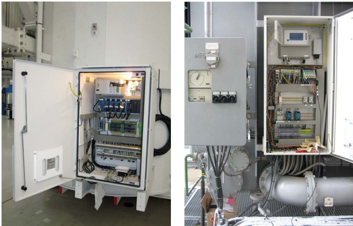
Fig. 7.43 Transformer monitoring with PD monitoring subsystem – Koncar (left), Alstom (right)
