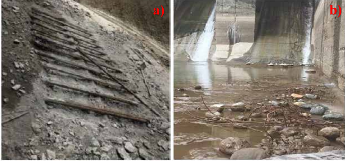
Figure 2 : Concrete abrasion over the spillway surface (a) stilling basin (b), DGPC (2021)
